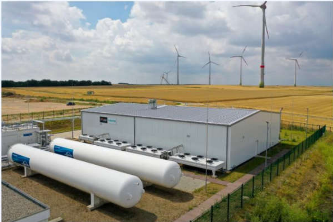
Figure 4: Wind turbines next to a green hydrogen facility in Mainz, Germany. (Picture Source: https://www.bloomberg.com/news/articles/2020-07-23/cheap-wind-power-could-boost-green-hydrogen-morgan-stanley-says )
