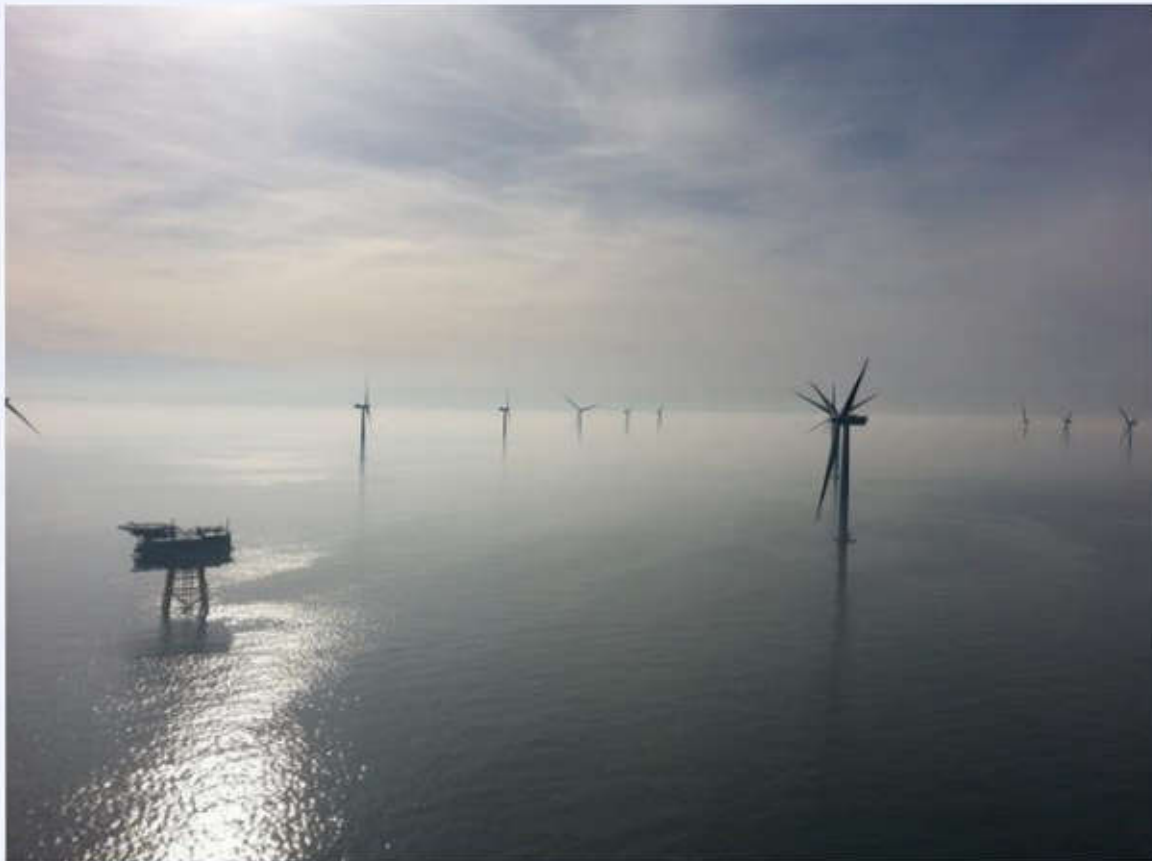
Figure 7: The Offshore Wind Farm Riffgat in the North Sea. (Picture Source: https://commons.wikimedia.org/wiki/File:Nebel,_Offshore-Windpark.png )
