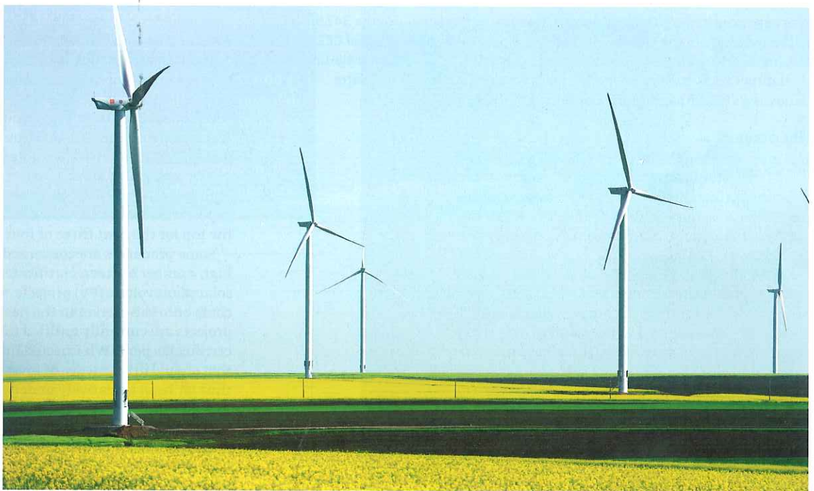
Being built CEZ's 600MW Fantanele-Cogaelac wind farm due for completion later this year
